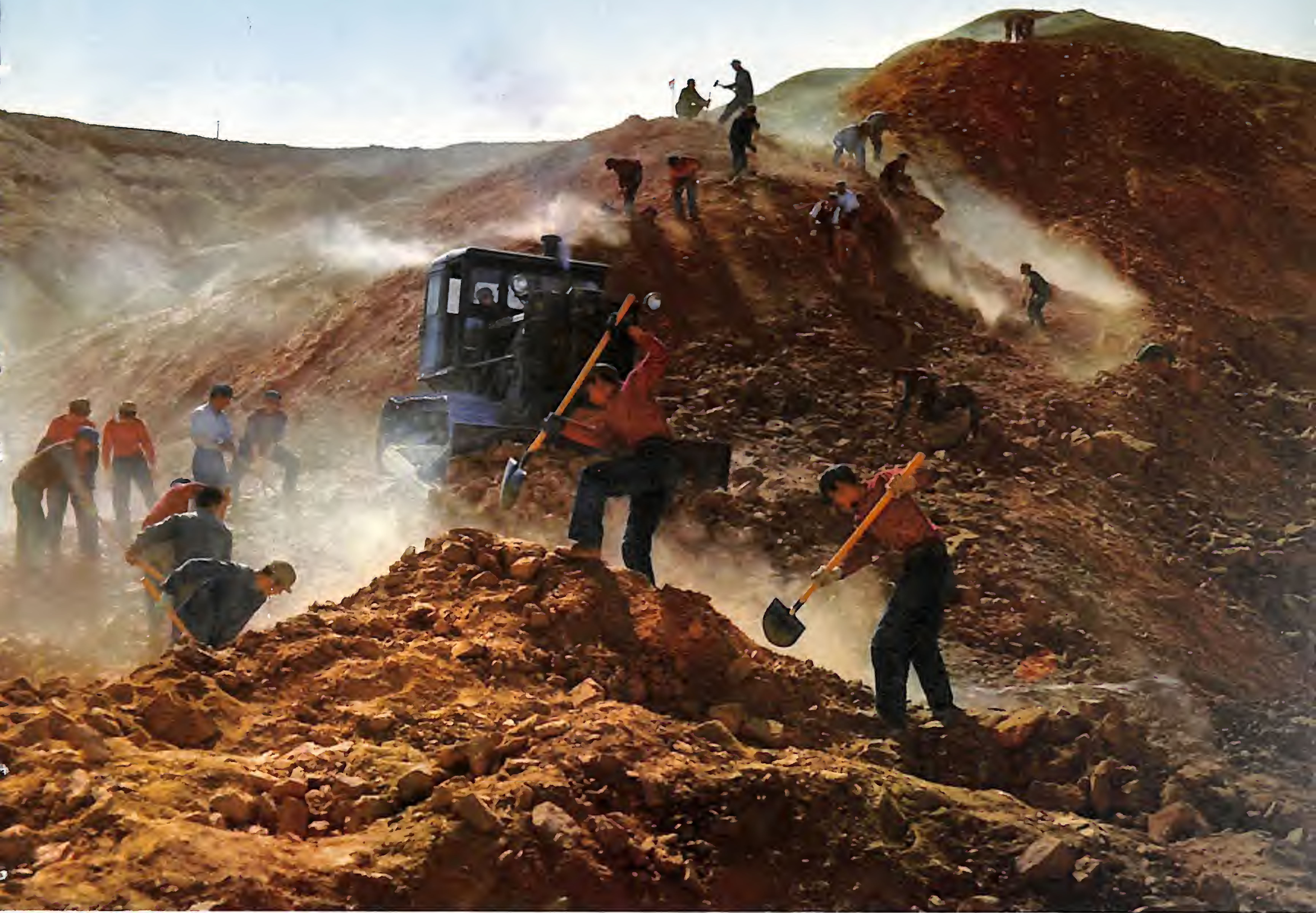
Making a road and levelling a drill site.
